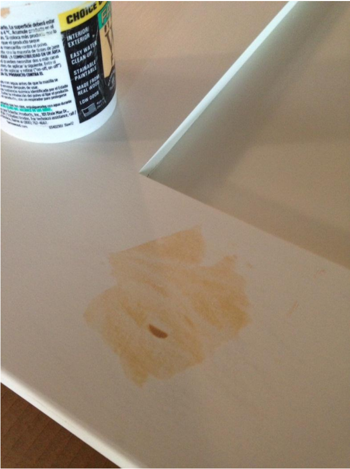
Picture 1: Filling in a small Dent. Note: Colored filler was used for illustrative purposes only.
